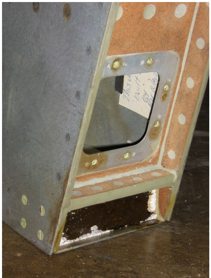
Photo 27: Exposed Root Base Channels
