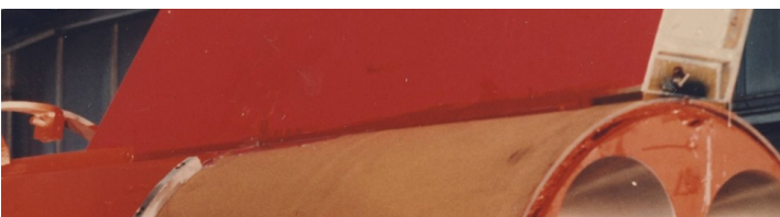
Photo 26: No Visible Rivets
